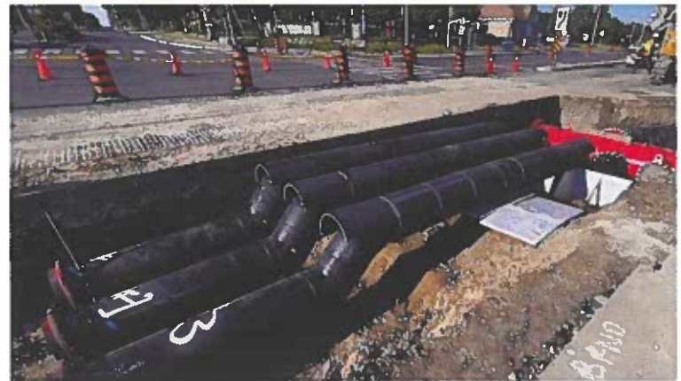
Temporary sewage bypass pipes along 16th Avenue
